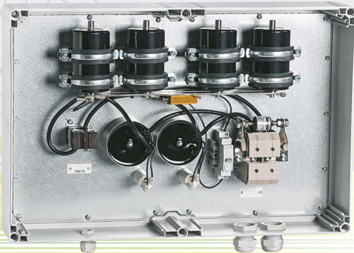
Leutron's protective devices are maintenance-free due to enclosed arresters
